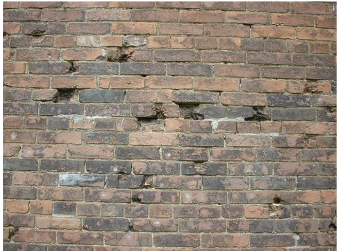
Same wall of the smokehouse, 2010.
